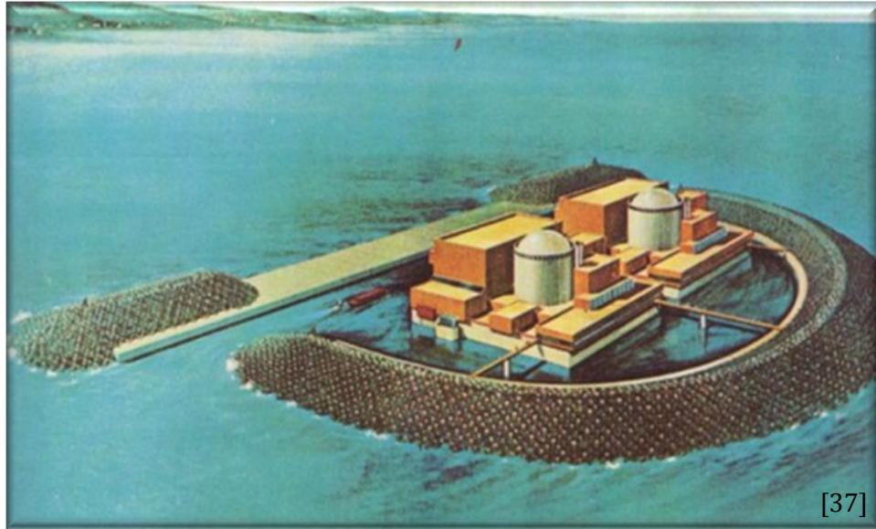
Figure 6.5 Offshore Floating Plant with Breakwater
